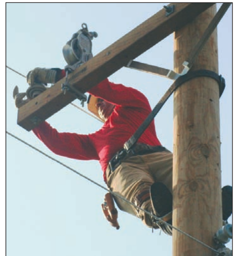
Eddie Bell, above, ties in a phase conductor to an insulator in the B1 Tie-In event, and Jeff Milam, below, ties in a neutral conductor to an insulator in the same event.
