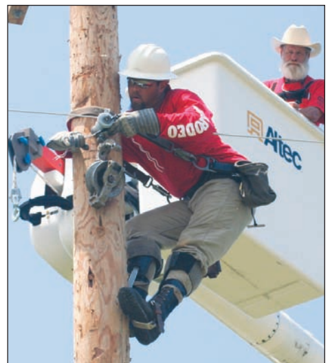
Eddie Bell, above, ties in a phase conductor to an insulator in the B1 Tie-In event, and Jeff Milam, below, ties in a neutral conductor to an insulator in the same event.
