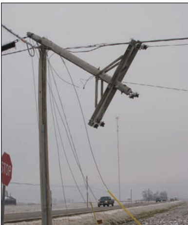
Ice and snow covered trees and power lines like a crystal blanket, so heavy that they snapped trees, distribution lines and poles.
