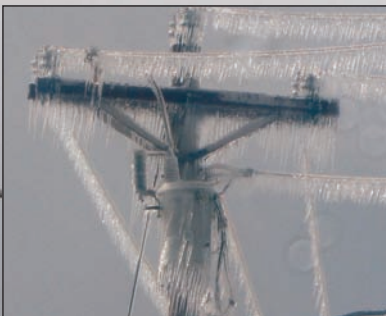
Ice and snow covered trees and power lines like a crystal blanket, so heavy that they snapped trees, distribution lines and poles.
